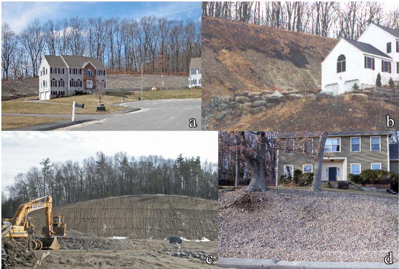
Figure 2. Drumlin modifications within the study area in eastern Massachusetts. A) An example of the large houses on relatively small lots associated with significant landform modifications. B) Slope failure on an excavated cut (Phillips Hill, Hudson). C) Large excavation of drumlin end (Indian Head Hill, Marlborough). D) Cut/fill slope on house lot (Jericho Hill, Marlborough). doi:10.1371/journal.pone.0046702.g002
