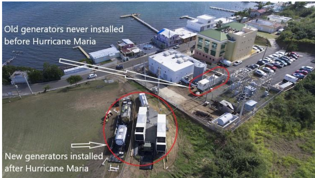
Figure 1.8 – Culebra’s Substation After Hurricane Maria with Old and New Generators
