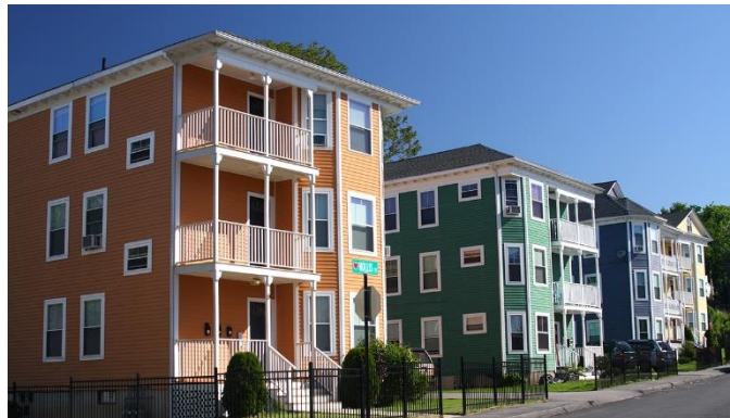
Figure 5: Renovated Triple-deckers in Worcester
