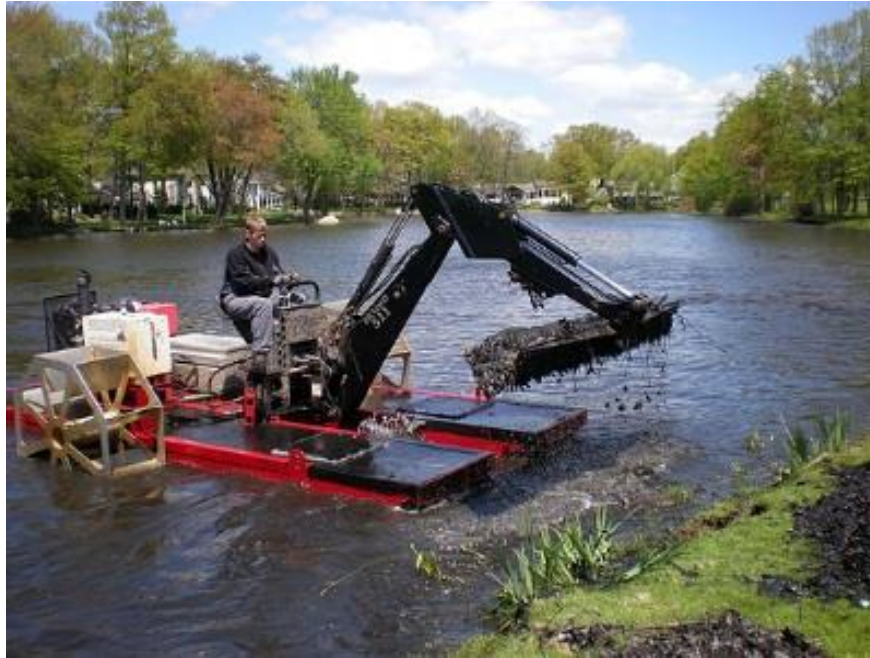
Figure 8. Hydro-rake unloading on shore. (Aquatic Technologies Inc., 2015).
