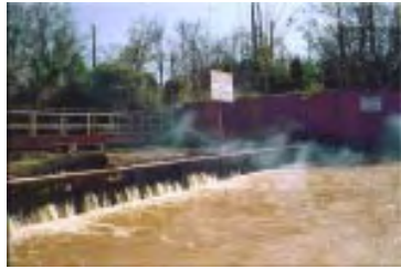
ORR wastes discharged from White Oak Creek into the Clinch River influence the environment over a half mile downstream.
