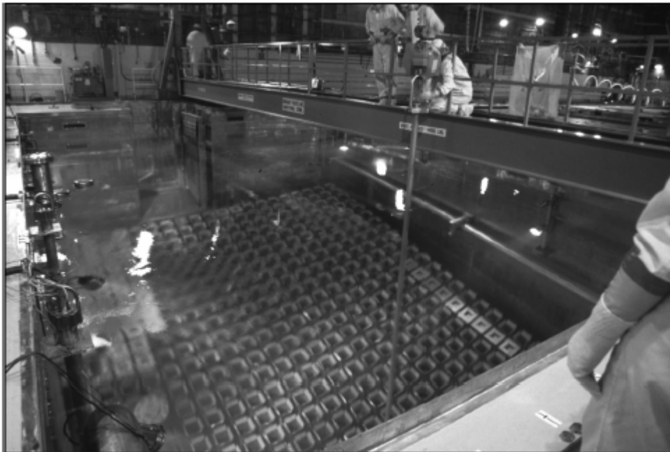
Source: Nuclear Energy Institute.
