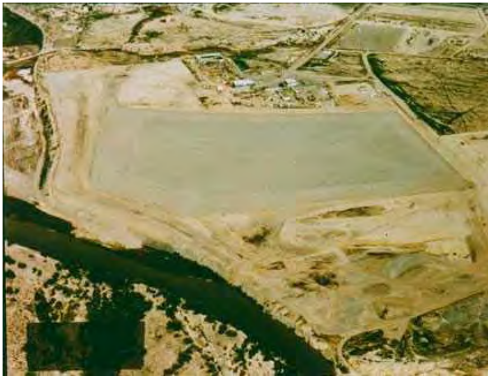
PHOTO 10 – Shiprock, NM UMTRAP following surface remediation in place, 1995
