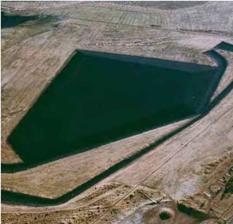
PHOTO 12 – Tuba City, AZ UMTRAP site following surface remediation in place, 1990
