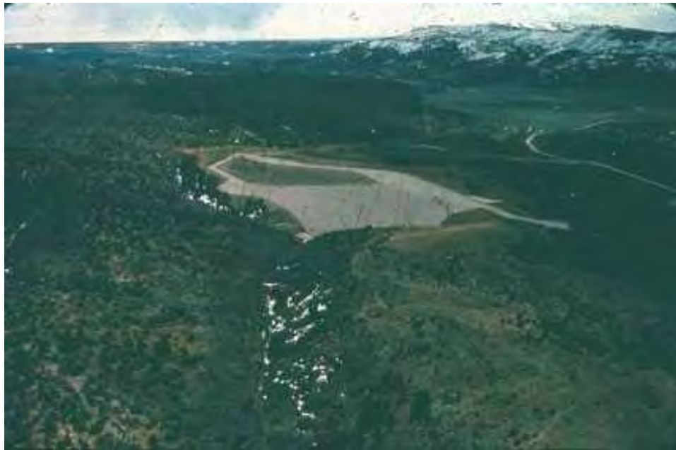
PHOTO 4 – Durango, CO UMTRAP site remote disposal cell at Bodo Canyon, 1992 Source: Paul Robinson
