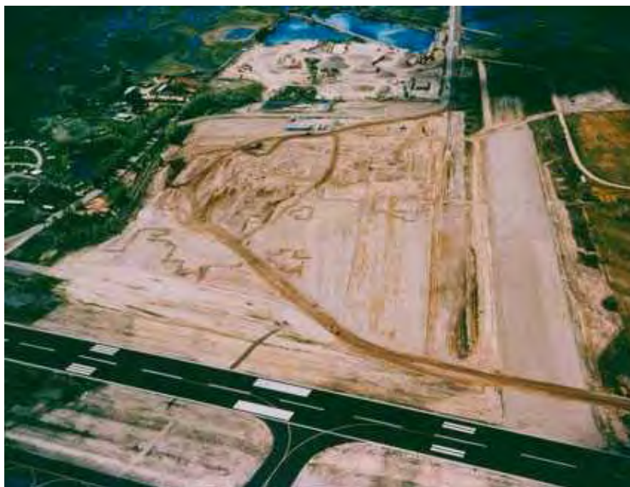
PHOTO 7 – Gunnison, CO UMTRAP Site prior to remediation, 1985
