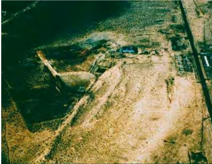
PHOTO 11 – Tuba City, AZ UMTRAP site prior to remediation, 1985
