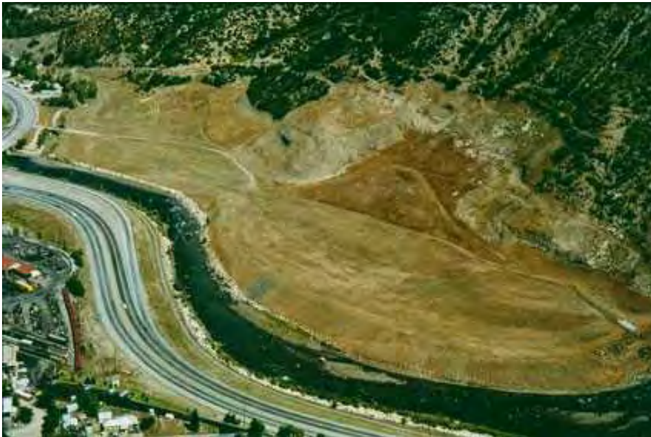
PHOTO 2 – Durango, CO UMTRAP Site after removal of all tailings, residual contamination and covering with radon barrier, 1991.
