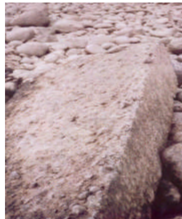
b. Close-up of concrete block.
