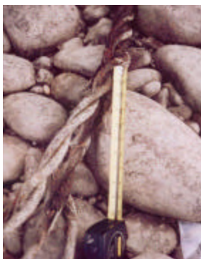
c. One-and-a-half inch steel cable.
