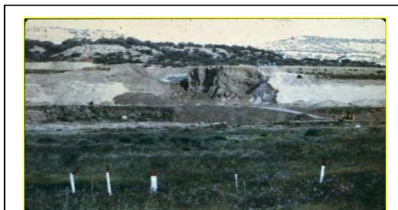
Figure I.2b. The breach in the tailings dam was clearly visible in this photo taken a day after the spill on July 16, 1979. SRIC photos by Paul Robinson.
